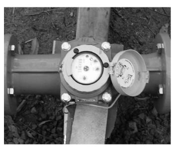
Select a water meter that is designed to read the amount of water flowing through the pipes and the operating conditions (such as temperature). Water meters are designed to measure flow within ideal ranges. Make sure you know and calculate anticipated peak flows and take this information when you see your supplier. Check that the water meter can meet both the minimum and maximum flow demands. There should be a tap installed next to the water meter to control the water flow when needed.
