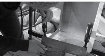
**Step 4:** Pop rivet the tabs which have been bent UP to the edges that they overlap as indicated by the blue dots in the diagram at the top of the page. These edges hold the box into shape.
