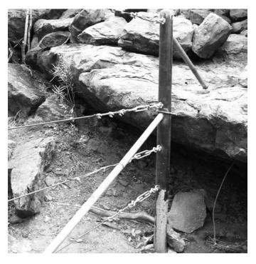
Use 8mm galvanised cable. The cable is threaded through the holes in the fence and either attached to the posts (simply with a bolt and a nut eyelet attachment) or can be fixed to rock using a threaded rod and chemset glue. Short lengths of cable can be tensioned with a large turn buckle, but larger lengths may need to be tensioned using a kangaroo jack or hand winch.
