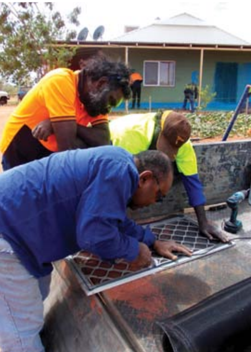
Above: Fly screen repairs at Utopia Homelands.
