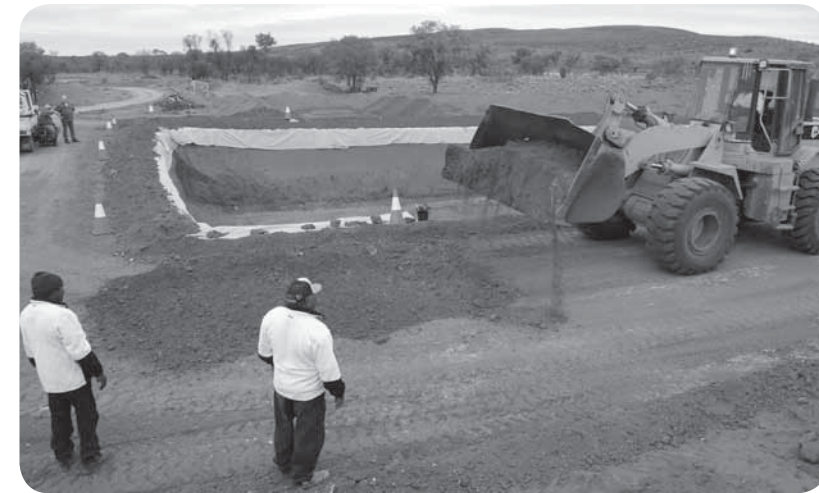
Tjuwanpa Tip under construction
