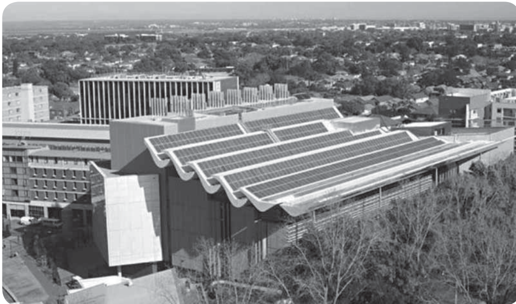
Tyree Energy Technology Building UNSW.
