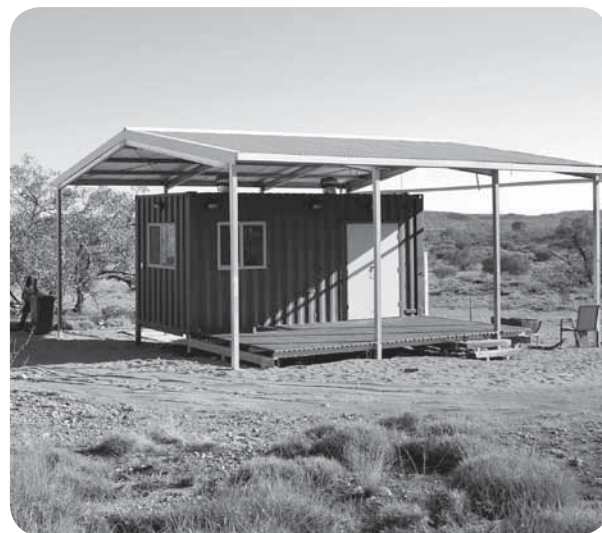
Re-fitted shipping container at Urremerne.
