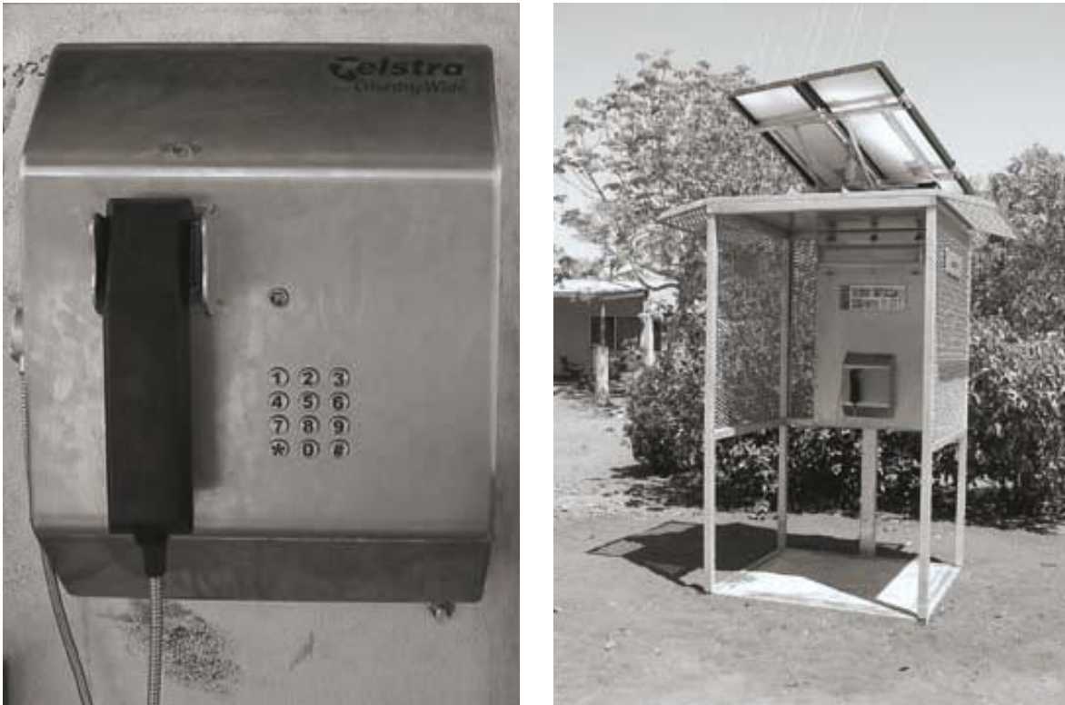
Figure B6.3: Community phone and installation in a remote area cabinet
