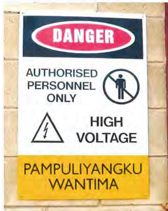
Image 3: Danger sign in language, Oak Valley Power station. Bushlight recommends the use of a safety theme in ongoing education programs.
