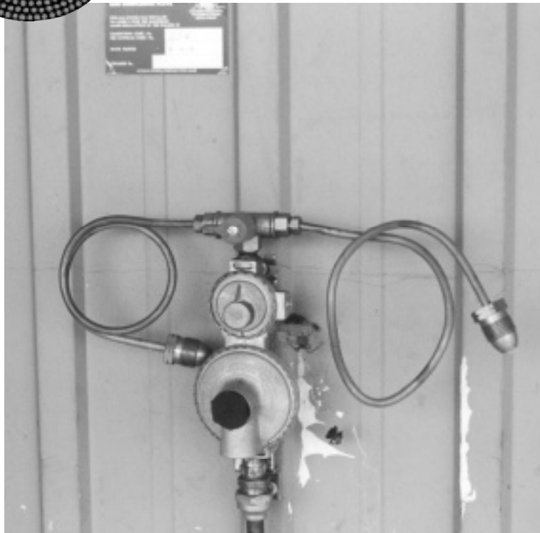
THE RIGID COPPER PIG TAIL IS EXPERTLY AND INEXPERTLY BENT INTO SHAPE (LEFT). WITH THE USER-FRIENDLY, FLEXIBLE PIG TAIL FITTING (ABOVE), THE REFILLED GAS BOTTLE NEED NOT BE PUT BACK IN EXACTLY THE SAME PLACE.
