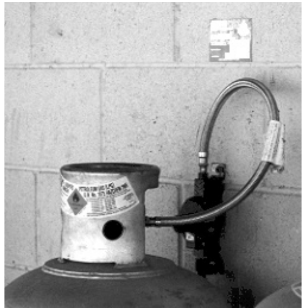
THE RIGID COPPER PIG TAIL IS EXPERTLY AND INEXPERTLY BENT INTO SHAPE (LEFT). WITH THE USER-FRIENDLY, FLEXIBLE PIG TAIL FITTING (ABOVE), THE REFILLED GAS BOTTLE NEED NOT BE PUT BACK IN EXACTLY THE SAME PLACE.
