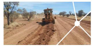
Training with Central Land Council included Grader machine check, identification of hazards and environmental issues, managing soil erosion through moving and bringing soil into the gully to be filled and levelled off, and grader operation.
